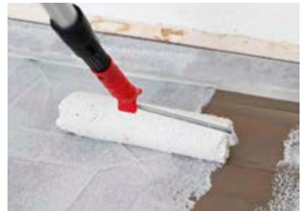
3| Secure edging strips and prime
