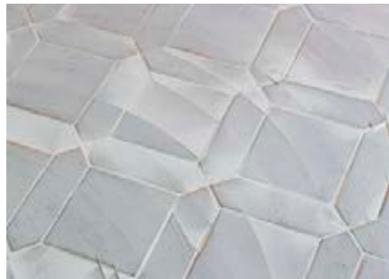
2| Smooth out the joints with screed
