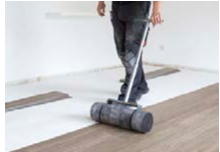
6| Roll to ensure even application of adhesive
